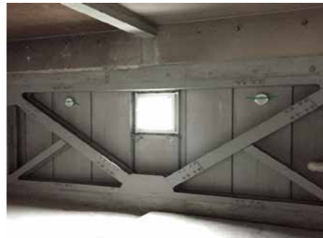
Bracing of frames inside the structure
