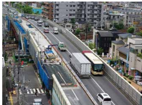
Deck slab replacement
