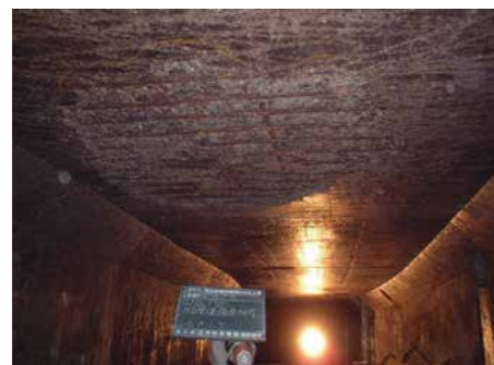
Sewer pipe before renewal
