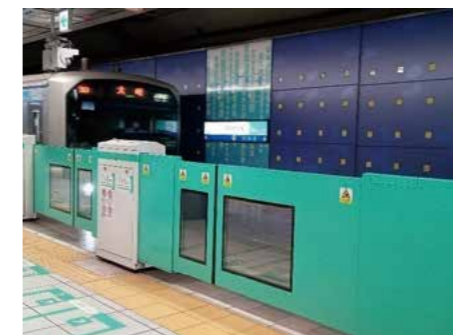
Platform door installation status 48%
