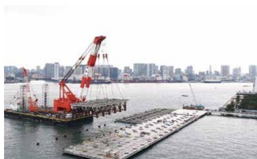
Using the jacket method to construct earthquake-proof reinforced quays
