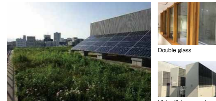
Solar power generation equipment / Rooftop greening
