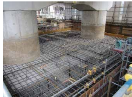
Pier foundation reinforcement
