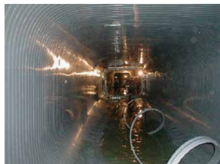
Sewer pipe during renewal
